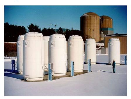
Figure 4: Current TN-40 and TN-40HT Casks on ISFSI Pad
