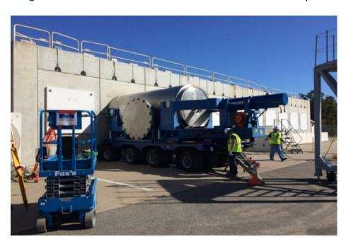
Figure 3: Placement of Canisters in Horizontal Concrete Overpack
