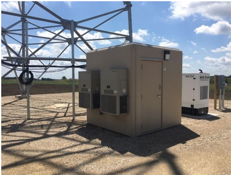
Figure 7 Typical Communication Shelter
