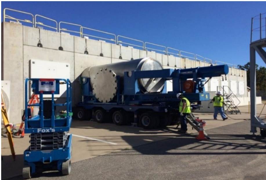
Figure 3: Placement of Canisters in Horizontal Concrete Overpack
