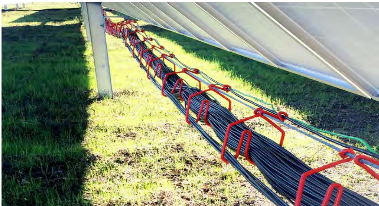
Image 1. Hanging Harness System for DC Cabling Between Panels and Inverters
