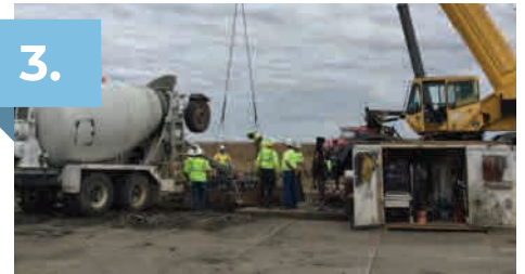
Foundation Drilling & Pouring
