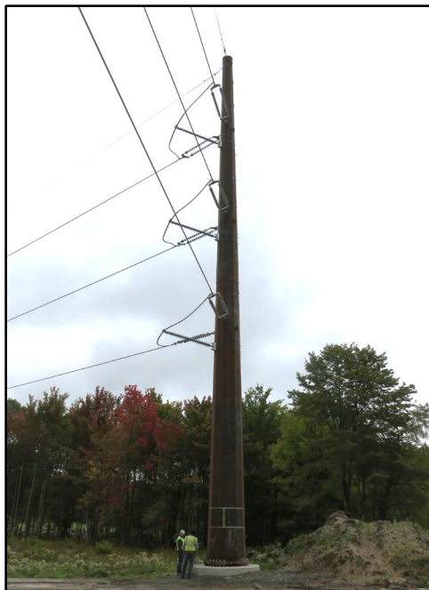
Image 2.5-2. Example 161-kV weathering steel monopole deadend structure in a single-circuit vertical configuration.
