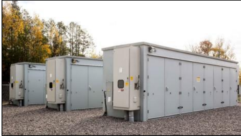
Image 3.1-6. Example self-contained energy storage system cabinet.
