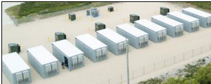
Image 3.1-8. Example self-contained energy storage system cabinet.
