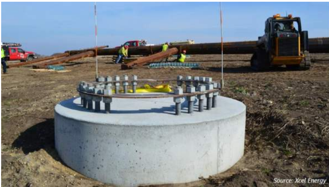
Photo 3-3 Finished Structure Foundation
