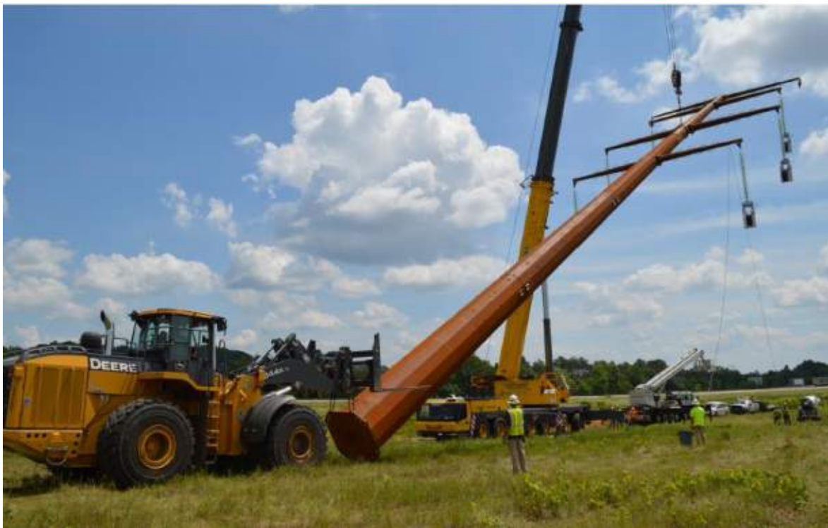
Photo 3-4 Erecting Structure with a Crane
