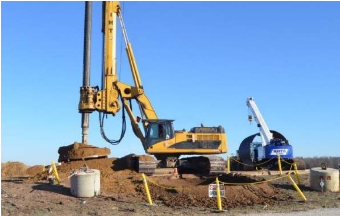
Photo 3-2 Drilling a Hole for a Structure Foundation
