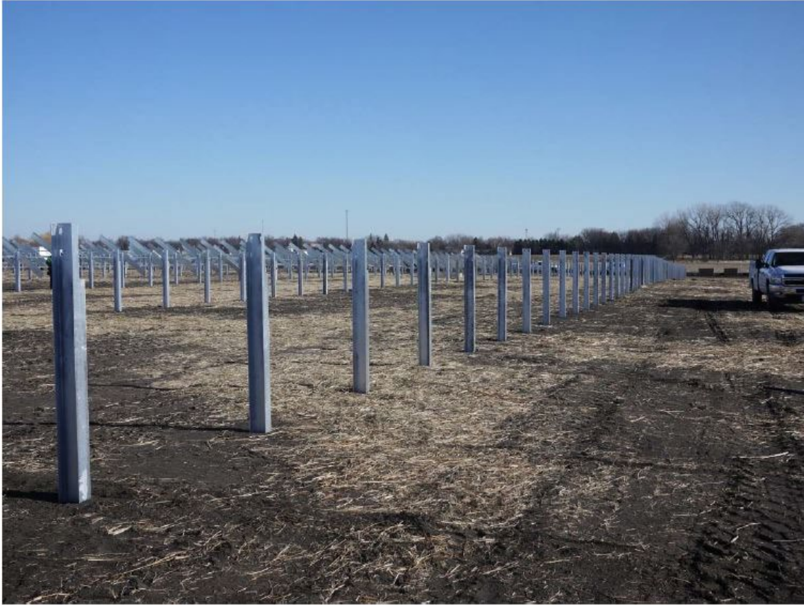
Figure 4.1.1-3: Standard Steel Pier Foundations
