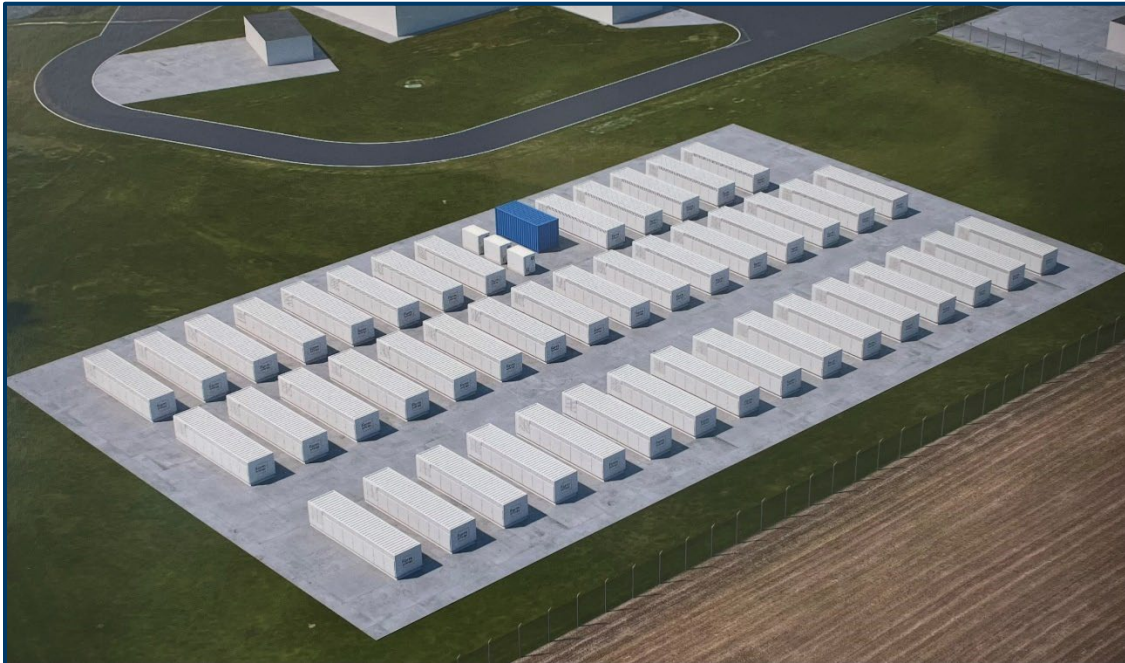
Figure 7 Energy Storage Project Visualization
