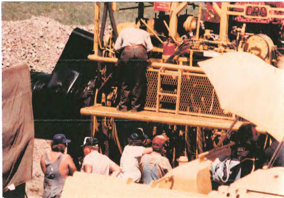
#16 Taping machine wrapping pipe with plastic tape to prevent corrosion. It was stalled at the time of the photograph.
