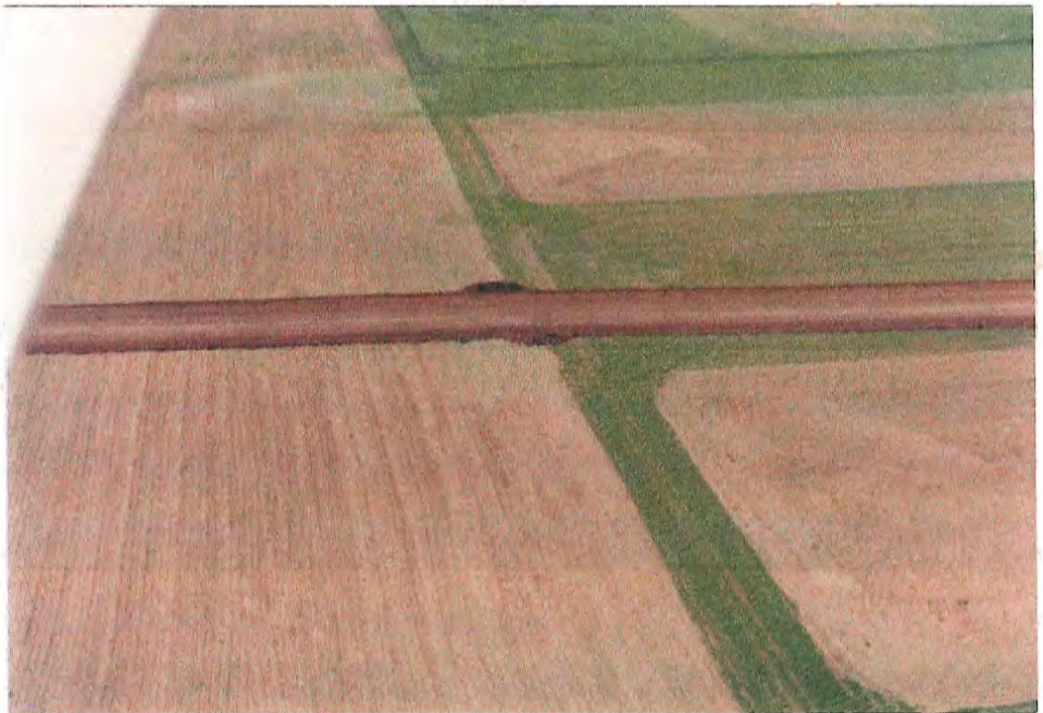
#52 An 85-foot cleared right-of-way on cropland in Roosevelt County on June 26. The r-o-w width increased slightly as the pipeline was constructed, but the width was well within 100 feet in most cases on this flat terrain.
