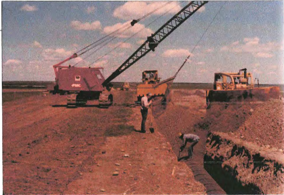
#19 Backfill operation consists of: augering, a dragline pulling in the rest of the ditch spoil, and a front-loader bringing up the rear acting as a packer. The man on the pipe in front of the auger is responsible for flipping rocks off the pipe to prevent damage to the wrap. Photo taken June 26 on state parcel PH012.
