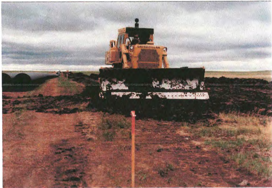
#5 Dozer blading 3-4 inches of topsoil from over trench area prior to ditching. This operation was combined with r-o-w clearing when the terrain was not as flat as shown in the photo, taken on July 16 on state land parcel VA057 west of the West Fork Procupine Creek.
