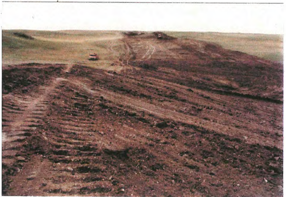
#78 Typical clean-up in progress in wide r-o-w area in Phillips County. Dozers first push the soil back roughly to the original contour, then a road grader with chisels reduces soil compaction and finishes contouring. Note that there has been extensive traffic outside soil/spoil storage areas. This adds to r-o-w width requirements as noted earlier. Photo taken July 22.
