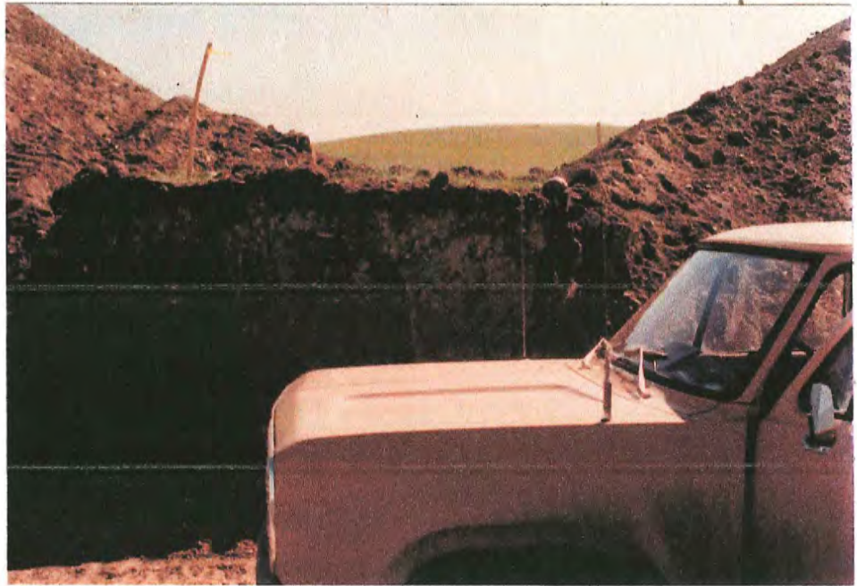
#64 Side-hill cut on work pad (as in cross section "A" on Figure 2) on state parcel PH026. This was the cut made in the hill on the other side of the drainage way shown in #63. Note the shallow depth of the A horizon (compare to #74 below.) Slope is about 7 degrees on this hill. Photo taken June 25.
