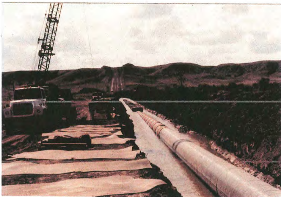
#30 Set-on weights being placed on pipe after it is in trench. Note the thick felt pads placed around the pipe to protect it. Photo taken July 14 on state parcel VA001.
