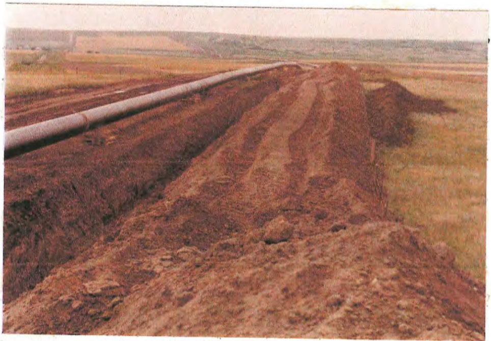
#79 State parcel R0142. Only the area shown in the photo is crossed by the pipeline. Note that the r-o-w was fenced but backhoe widening of the trench added material to the spoil pile, covering the fence and topsoil. The view looks northwest on July 24 from the southern edge of the parcel.
