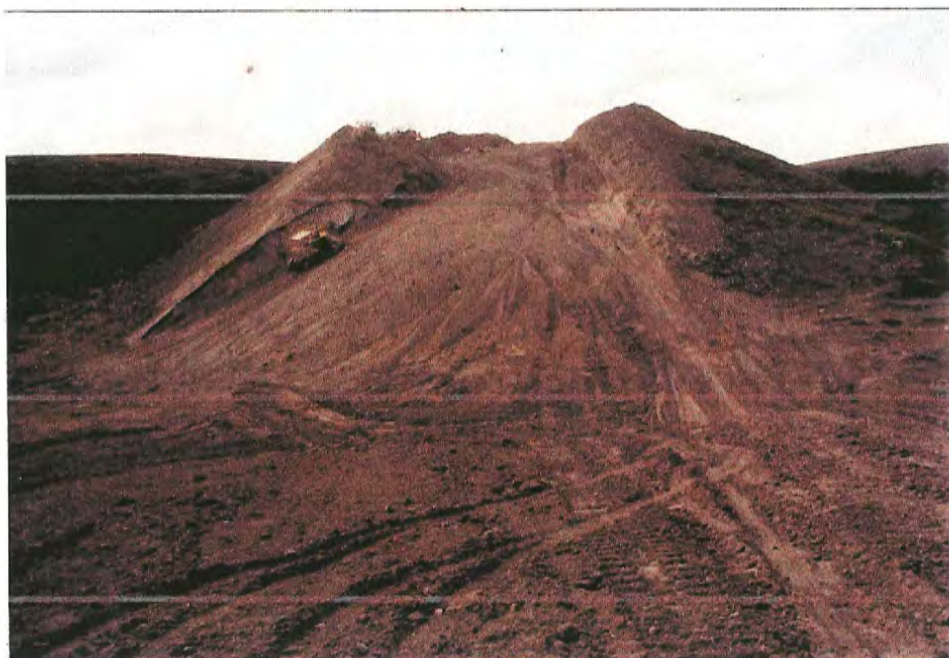
#22 West bluff of Frenchman Creek Valley being re-contoured on July 22. See photos #40 to #43 for a more detailed description of restoration on rough terrain.
