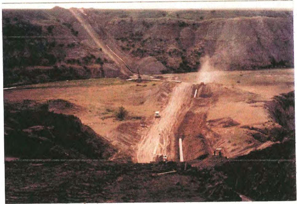
#38 Rock Creek Canyon, looking west on July 22, construction in progress. Note: 1) Dozer covering pipeline, 2) River section lying next to creek on the base of the west bluff. This was the roughest terrain encountered in Montana.
