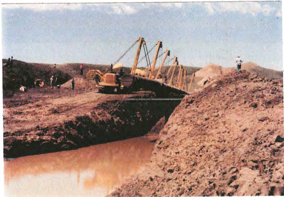
#34 Approaching the creek from the west. The lead tractor, not in the photo, has started to run out cable for pulling pipe. The foreman across the stream stands on the spoil bank to the right and orchestrates the movement of the tractors.
