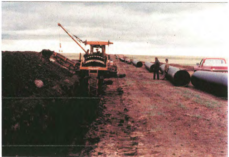
#8 Trenching on state parcel VA052 on July 16. Note the grass remaining on the work area. Terrain was flat and little side-hill cutting was required.
