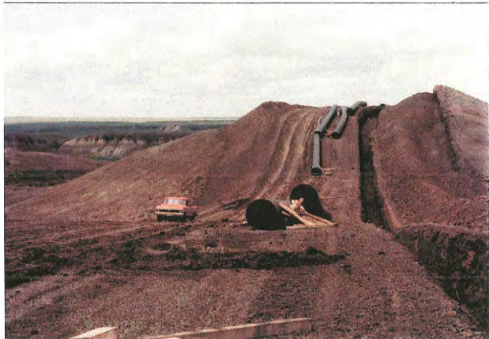
#44 Construction across badlands. The r-o-w crosses an unvegetated shale knob on the east side of the Bitter Creek Valley. The top of the knob was crossed rather than a drainageway because less erosion would occur on top. Note the depth of cut into the knob on the right side of the picture. Photo taken looking west on July 22.
