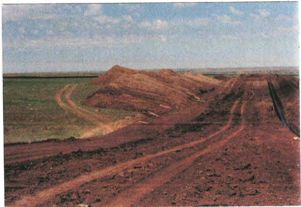
#59 Compare this view to views of cross section "A" on Figures 1-3. This photo, taken July 15, looks west on state parcel VA006. Note that there is poor topsoil separation in this area, although a small pile can be seen behind the large pile of subsoil.
