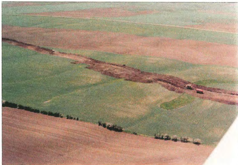
#4 Right-of-way clearing June 26. Soil and spoil is usually moved perpendicular to the centerline to simplify recontouring. All clearing was completed in Montana by July 15.
