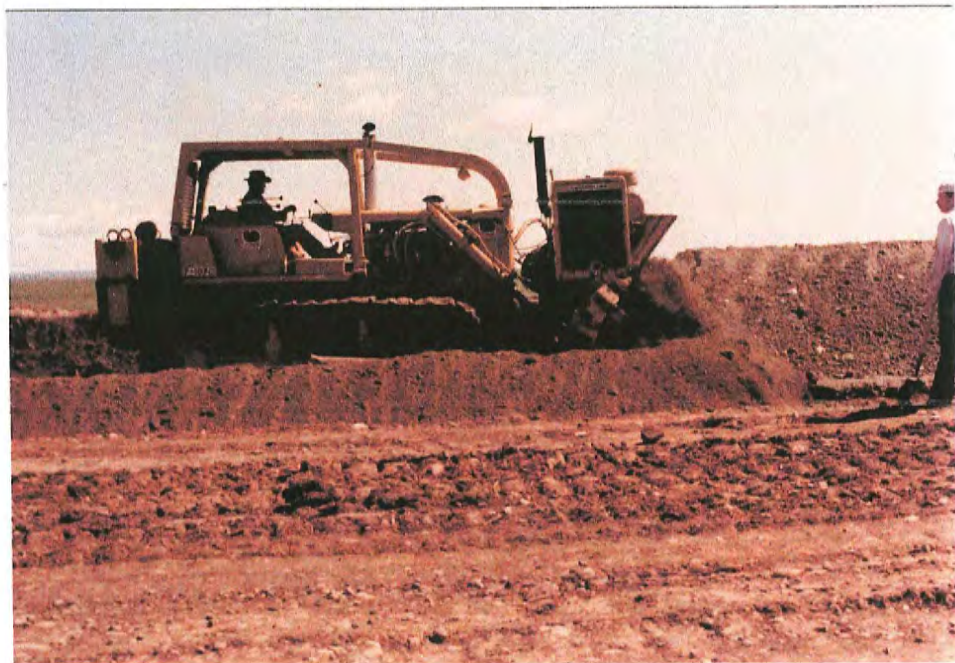
#18 Ditch spoil being replaced by auger mounted on front of tractor.
