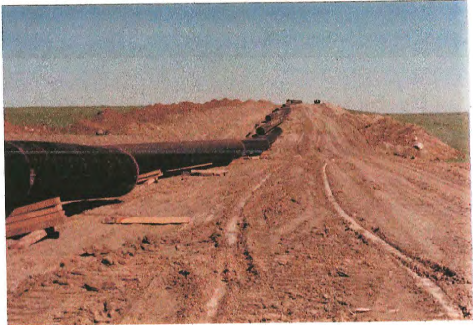
#58 Looking east on June 25 at a long stretch of south-facing slope on state parcel PH026. Note that on this parcel topsoil has been stored uphill to the left.
