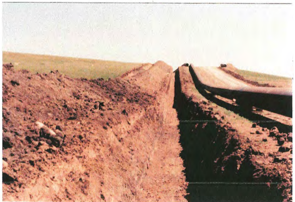
#55 Compare this view with that at cross-section "B" in Figures 1-3 (this view is to the east, however). Note the cut on the left providing fill for the work space on the right. This is taken about 1.5 miles west of state parcel PH018 near Turkey Track Road. Photo taken June 25.
