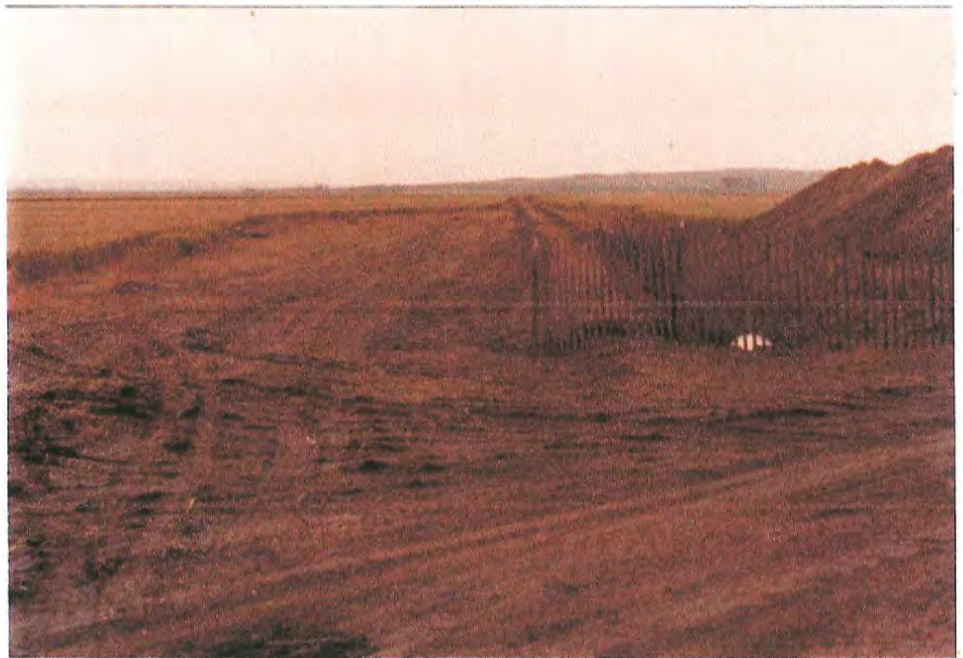
#54 Same view as #53 on July 24. This was the only state parcel that was cropped. The r-o-w was generally about 85 feet wide on this parcel although it was wider in the foreground because the field road was bored under rather than ditched through.
