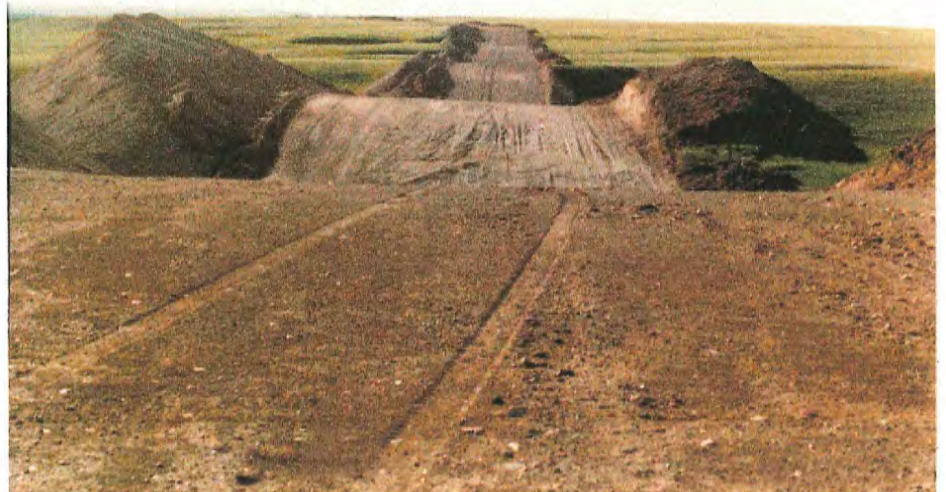
#70 Same view as #69, same spot, taken June 26, before ditching and pipe stringing began. Note that each ridge is cut extensively, resulting in more gradual bends on top of the hills. This result cannot be obtained at the bottom of drainageways, however, because the pipe cannot be placed in unconsolidated fill.
