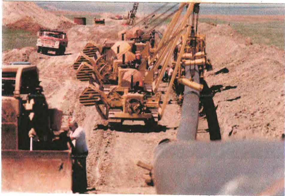
#15 Side-boom tractors lifting pipe and feeding it into the tape machine behind them. The tractors move slowly forward and the pipe is suspended on rollers. After wrapping, the pipe is lowered into the trench. The tractor in the foreground pulls a cart which carries hardwood blocks that prop up the welded pipe. This is state parcel PH012 on June 26.
