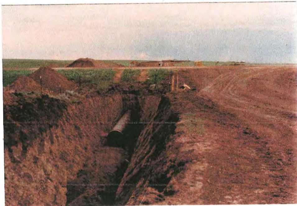
#47 Bored road crossing, Valley County. Boring was done, even on small roads, to prevent road maintenance problems. Photo taken June 23.
