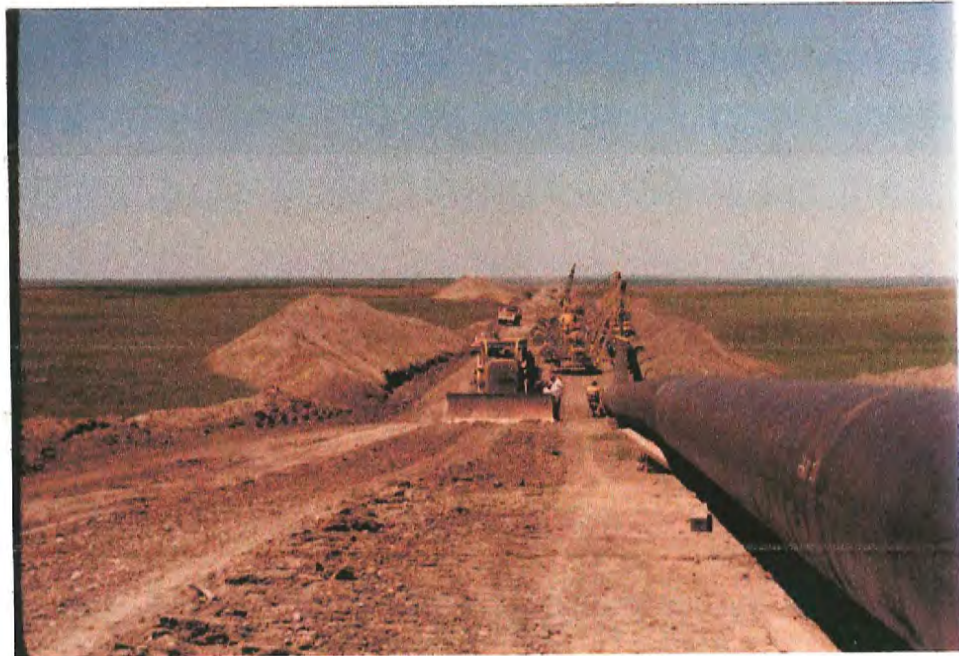
#62 Same view as #61 on June 26, and see view "A" on Figures 1-3. Note the lack of topsoil storage piles. This section was cleared in the first few days after construction began, and little topsoil was saved even though saving 12 inches of "topsoil" was stipulated on the Department of Lands lease. (See conclusions section.)
