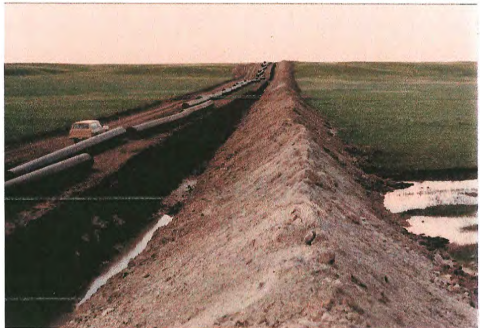
#51 Same view as #50, about 300 yards farther west and from atop the trench spoil bank on July 23. Note that in the distance a trencher was used and in the foreground a backhoe was used. An 85-foot right-of-way was cleared in this area, and it became slightly wider after ditching, especially where the backhoe was used.
