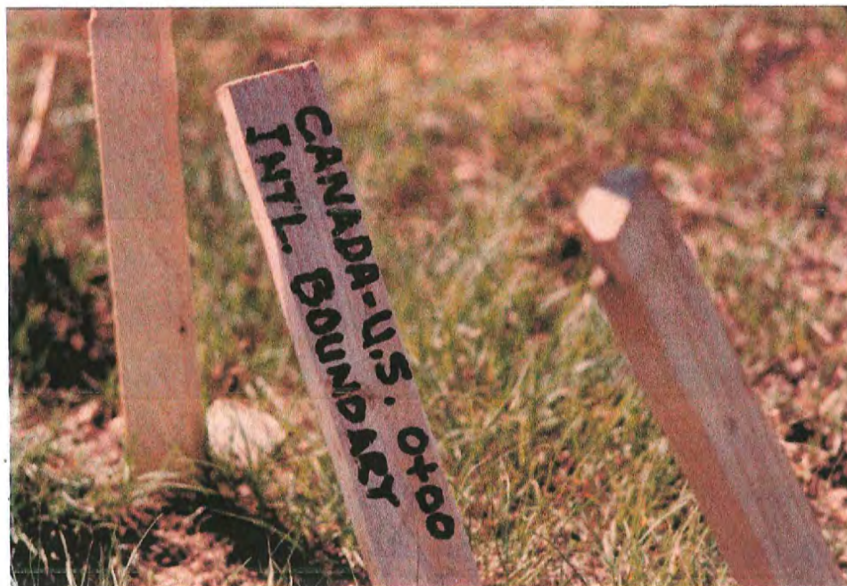
#49 Survey stakes along the r-o-w. Locations are given in the format "0+00". Table 1 gives survey stations for points where the pipeline enters and leaves state lands.
