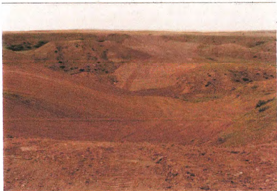
#43 Same coulee on July 22, from approximately the same spot as #42, after re-contouring. Waterbars, small dikes built across slopes to slow water erosion, are present but not visible.
