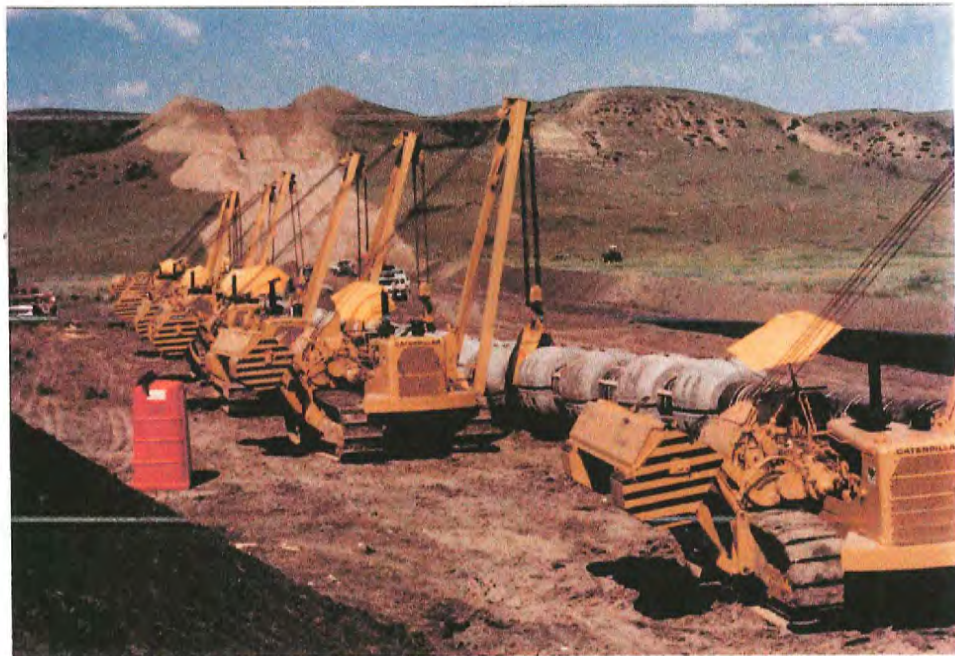
#32 Side-boom tractors lifting the creek section to pull it across. Concrete weights in place. The lead tractor, which winches the section across the creek with a cable, is in the foreground.
