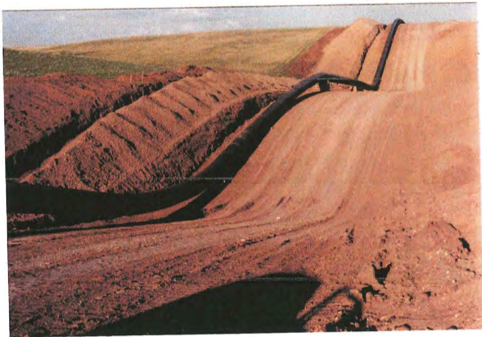
#13 Welding completed, and pipe ready for wrapping and lowering-in in Phillips County.
