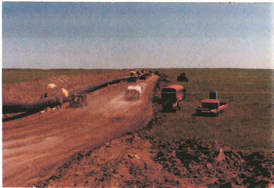
#11 Welding spread in Phillips County on state land parcel PH018 near Turkey Track Road. Photo taken June 25. Note the welding trailers at each weld. The farm tractor on the right side of the r-o-w was used to pull the trailer. The bus was used to bring pipeliners to work. It was about a 1.5 hour one-way trip to this work site from Glasgow.
