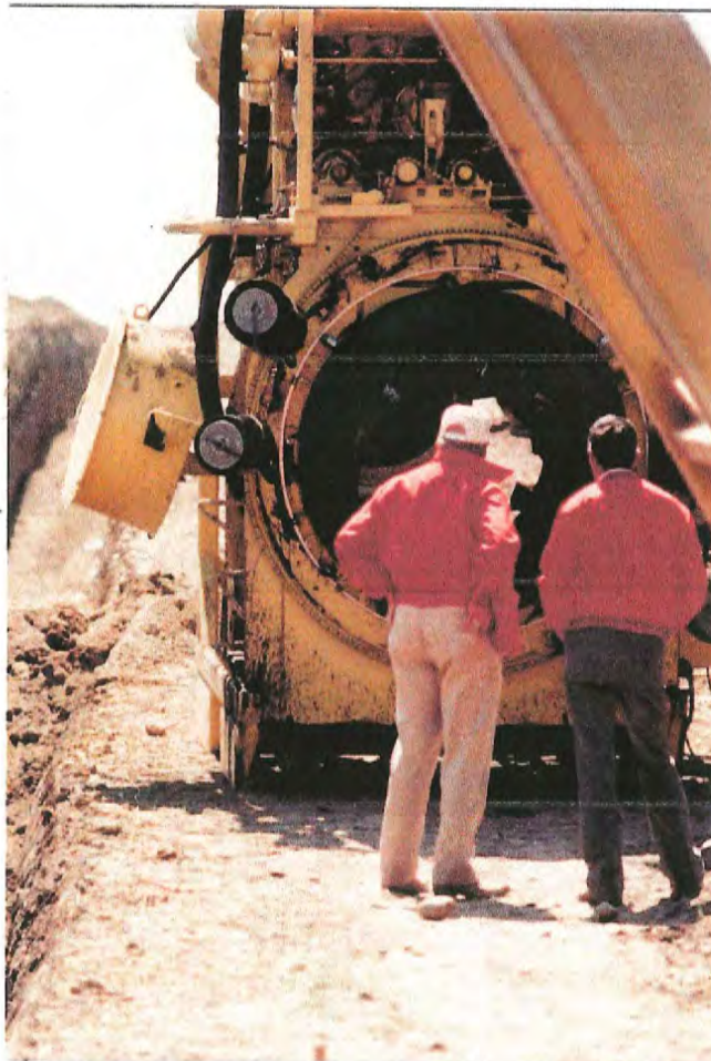
#14 Taping machine. In operation, it is suspended by a side-boom tractor. Pipe was coated with Teflon on the Western Leg of ANGTS rather than being wrapped with tape (see photo #9).
