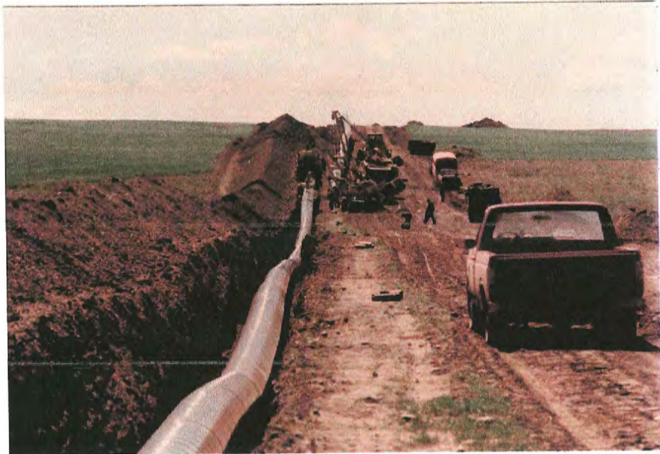
#17 Taped pipe after lowering-in, ready to be covered. Photo taken June 26 on state parcel PH012.
