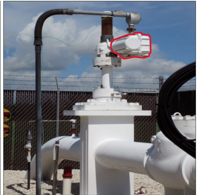
Figure 3: A Hand Wheel Used to Close a Manual Valve (Outlined in Red on Left) and an Actuator Used to Remotely Close an Automated Valve (Outlined in Red on Right)
