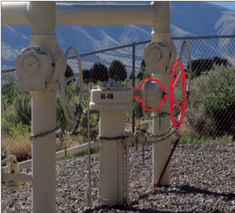
Figure 3: A Hand Wheel Used to Close a Manual Valve (Outlined in Red on Left) and an Actuator Used to Remotely Close an Automated Valve (Outlined in Red on Right)
