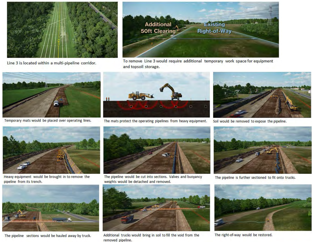
Figure 3-1: Stages of Pipeline Removal
