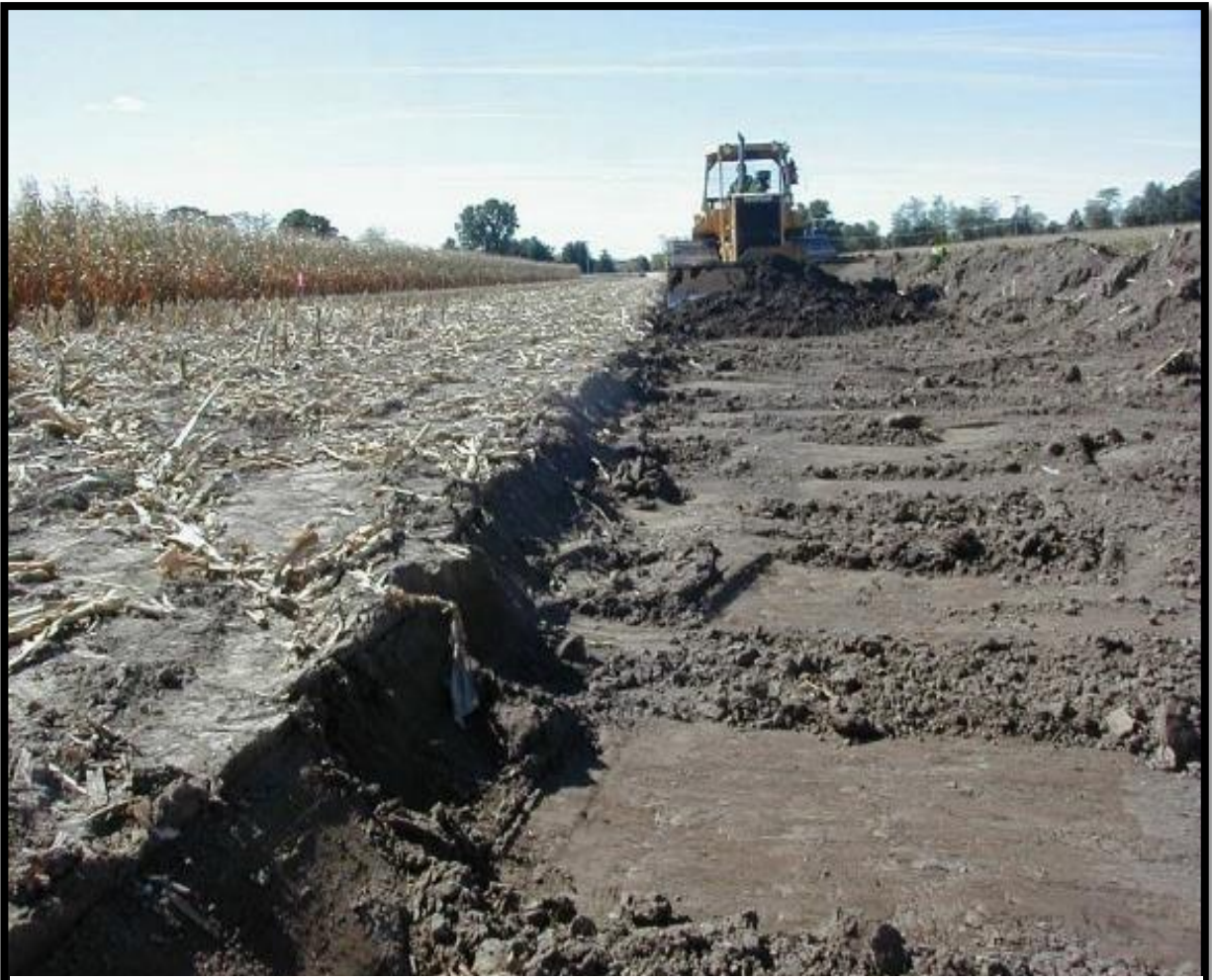
Figure 5.2.3-1: Topsoil Segregation
