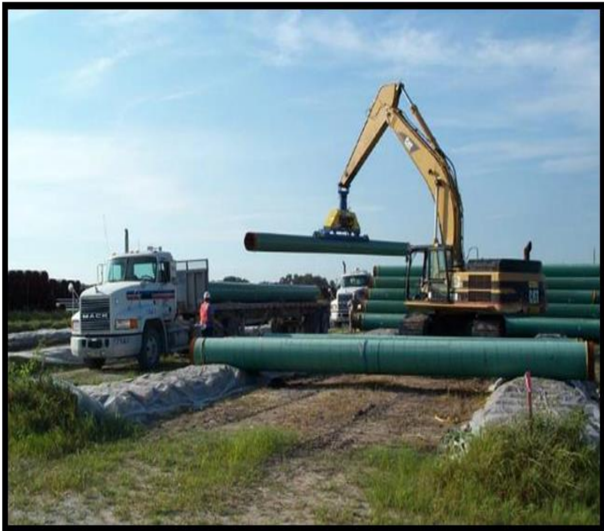
Figure 5.2.4-1: Pipe Loading
