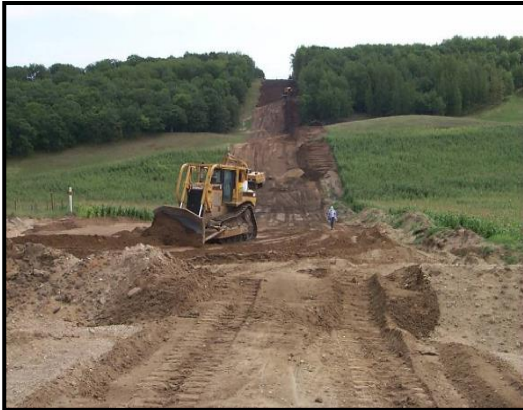
Figure 5.2.9-1: Regrading
