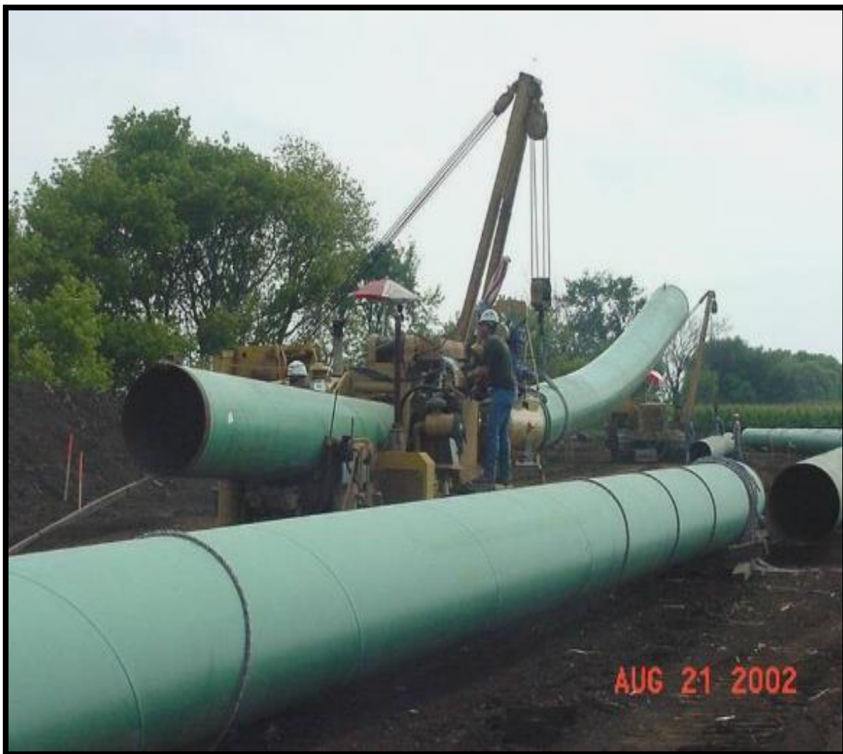
Figure 5.2.5-1: Field Bending
