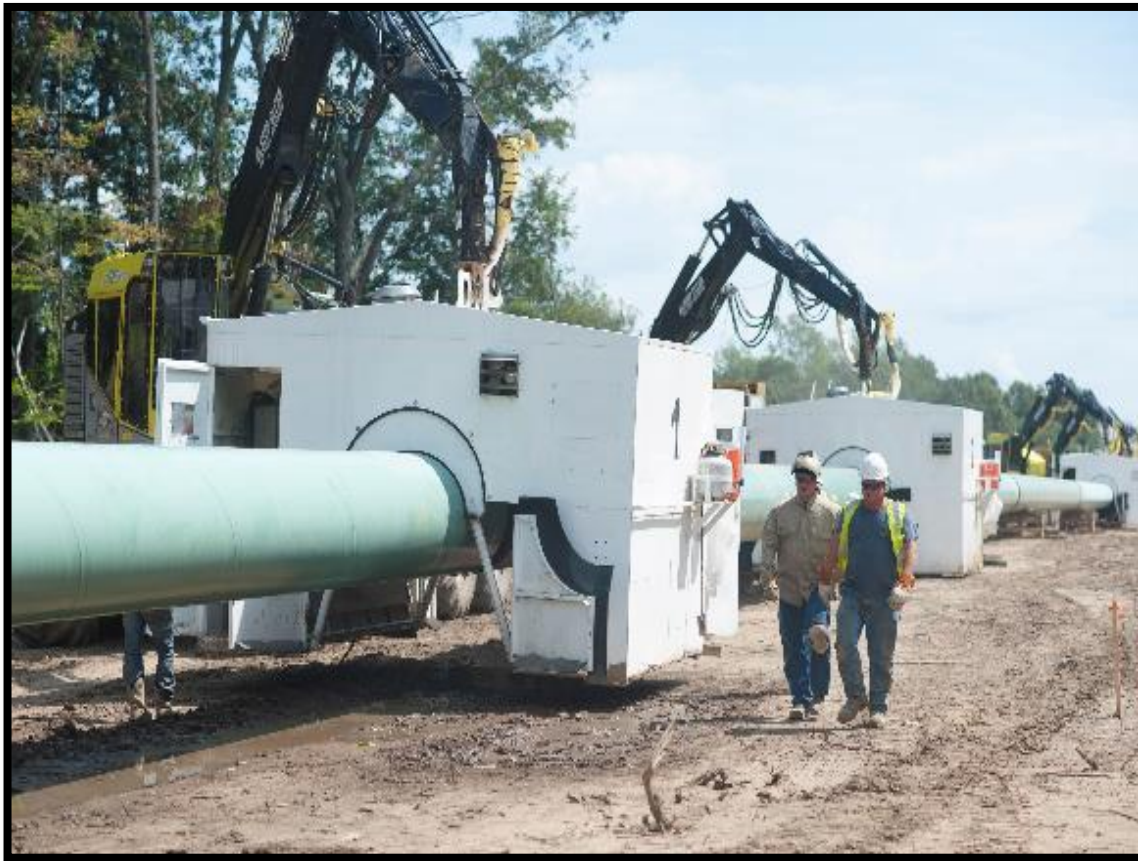
Figure 5.2.5-2: Welding Shacks
