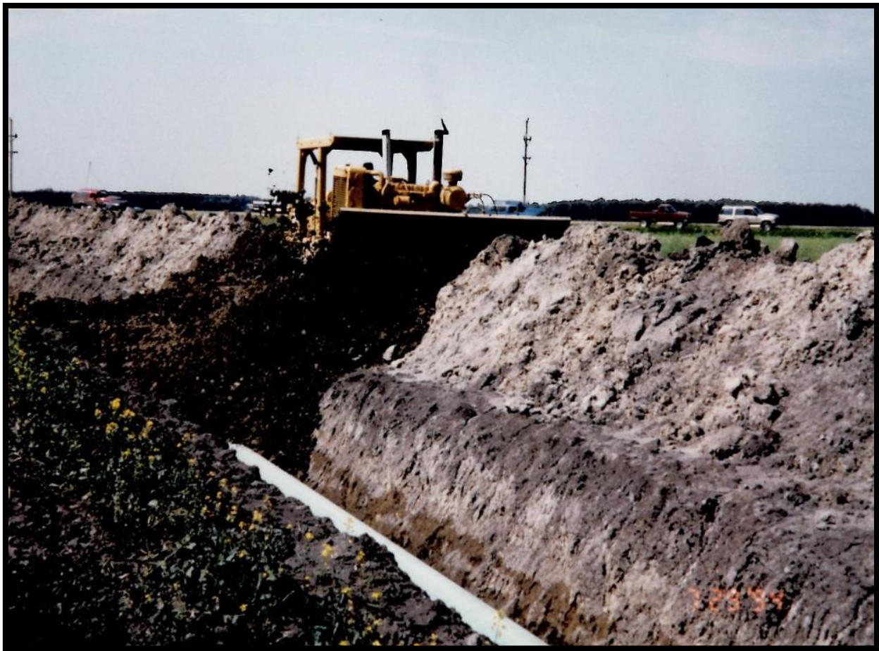
Figure 5.2.7-1: Backfilling
