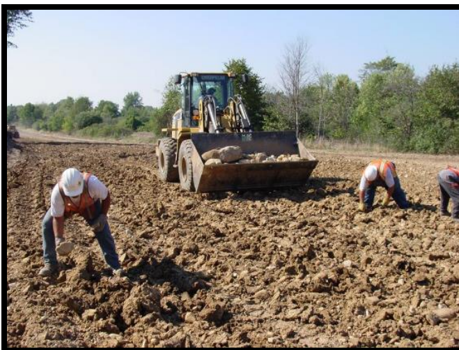
Figure 5.2.9-3: Rock Removal
