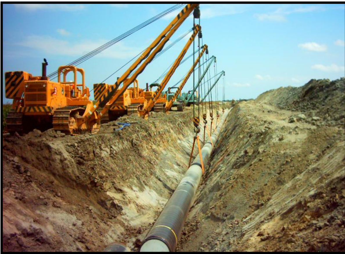
Figure 5.2.6-1: Lowering of the Pipeline
