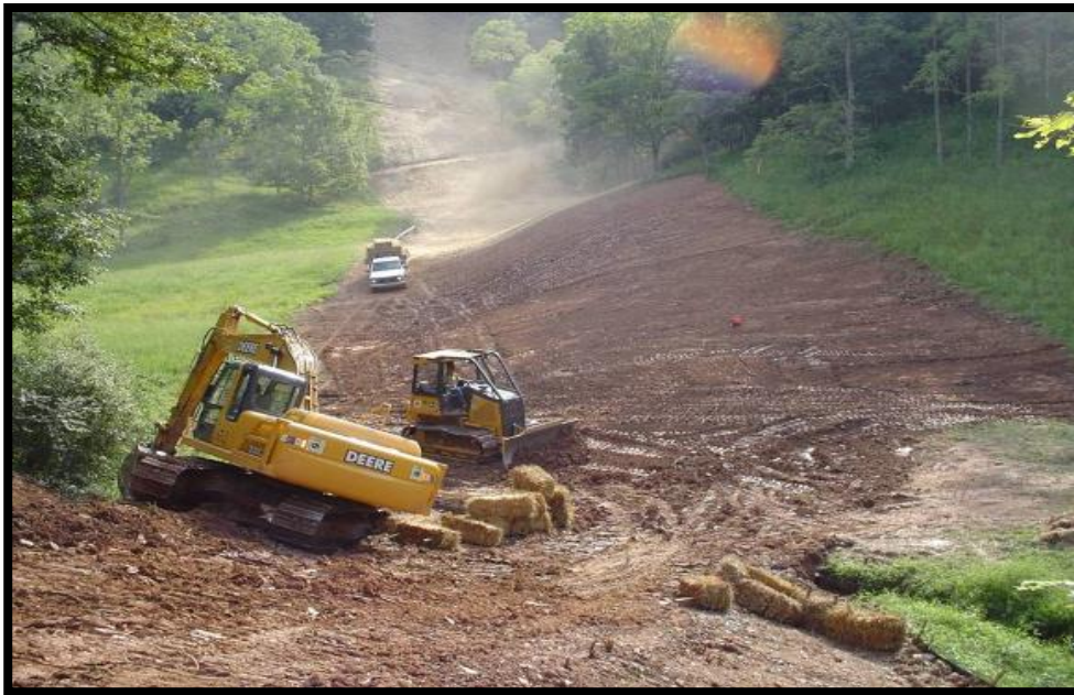
Figure 5.2.9-2: Erosion Control
