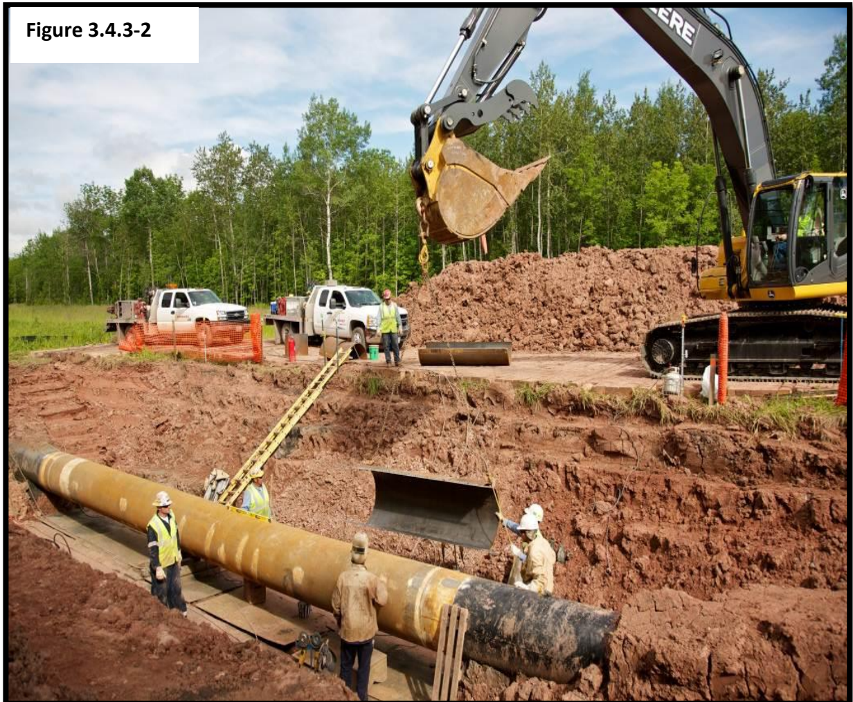
Figures 3.4.3-2: Placing a pipe sleeve on pipeline
