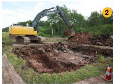
Excavate to expose the pipe
