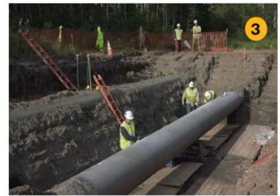
Clean the exposed pipe
