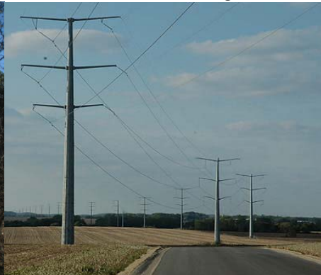
345 kV Transmission Line, Single Metal Pole
