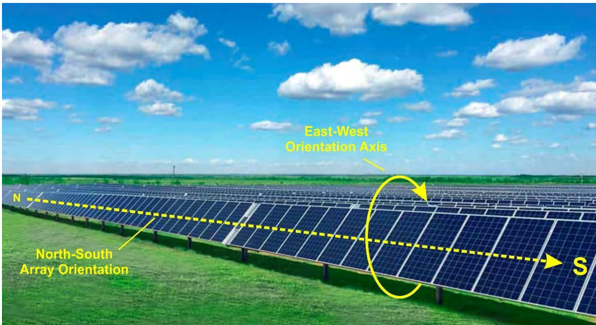
Figure 9 – Diagram Showing Tracker Array Rotation and Orientation for the Proposed Project
