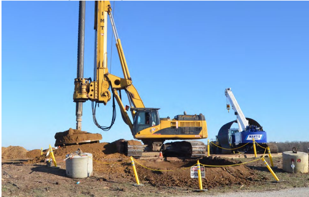
Diagram 3. Drilling a Hole for a Structure Foundation
