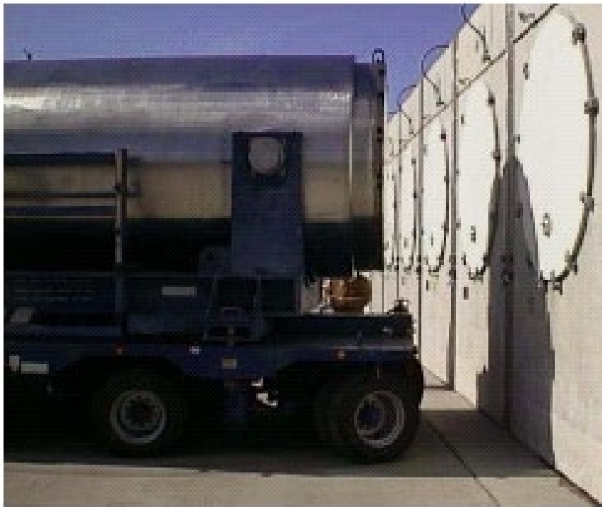
Figure C-9: Alignment of Transfer Cask with Storage Module
