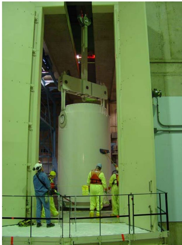
Figure 5. TN-40 Cask Removed from Spent Fuel Pool
