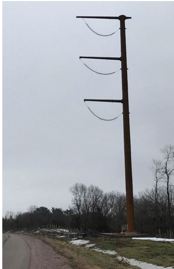
Diagram 12. Example: Single-Circuit Monopole 345 kV Structure 71
