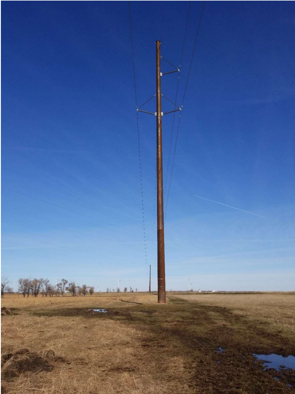
Illustration 1: Representative 161 kV Delta Configuration Single Circuit Structure Sample Photograph
