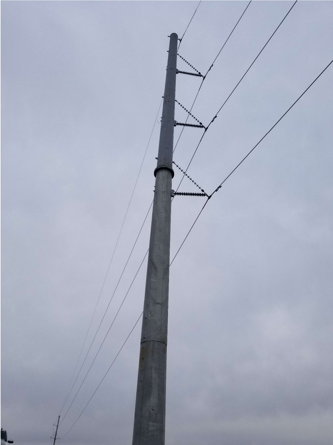
Illustration 2: Representative 161 kV Vertical Configuration Single Circuit Structure Sample Photograph
