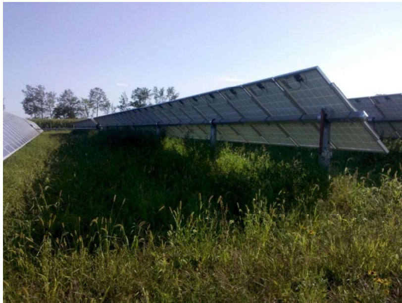
Image 1: Typical Solar Tracker Row Design
