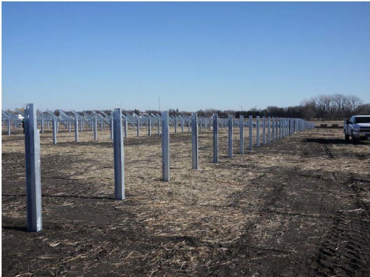
Image 2.2-4: Standard Steel Pier Foundations
