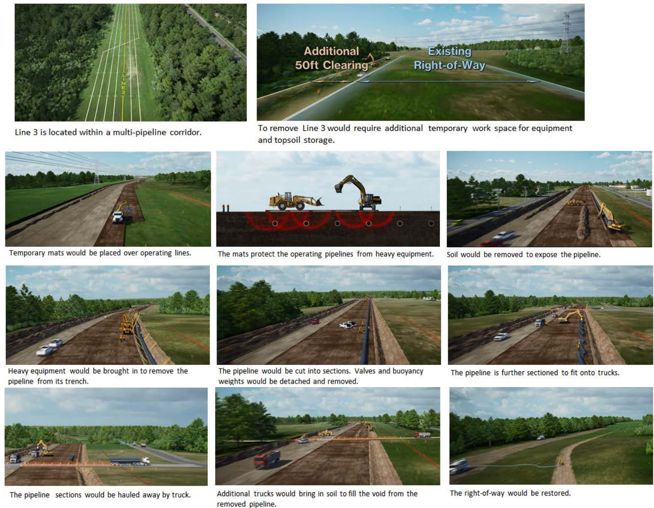
Figure 3-1: Stages of Pipeline Removal
