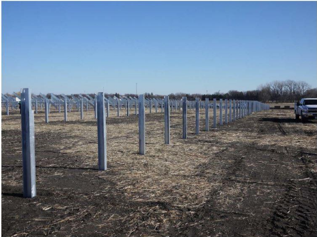
Image 4: Standard Steel Pier Foundations
